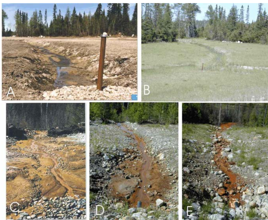
Figure 9 A) View of drain Cal-1 output, May 1999. B) Idem, but in June 2001. C) View of drain Dol-3 output, May 1999. D) Idem, but in June 2001. E) View of drain Dol-1 output, June 2001. Notice the iron hydroxides precipitates in the trenches.
