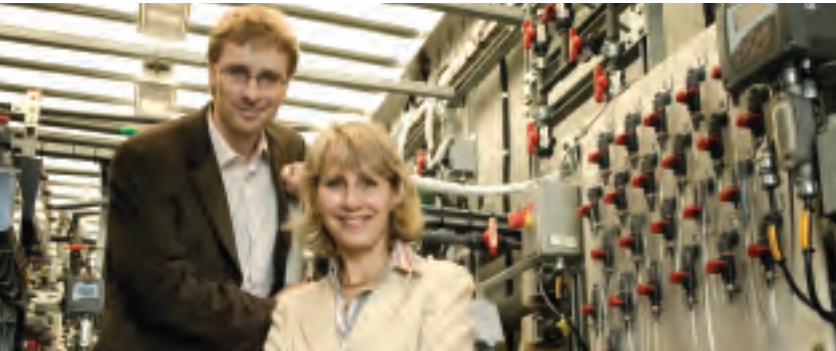
Benoit Barbeau and Michèle Prévost inside the mobile treatment unit.
